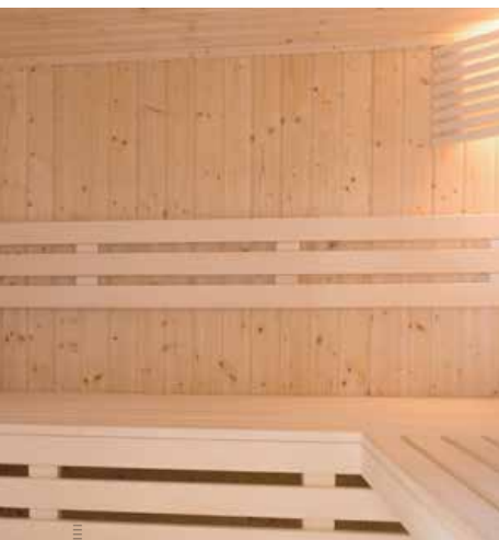
Nordic spruce as interior cladding, combined with straight, simple sauna benches in light, knot-free aspen.
